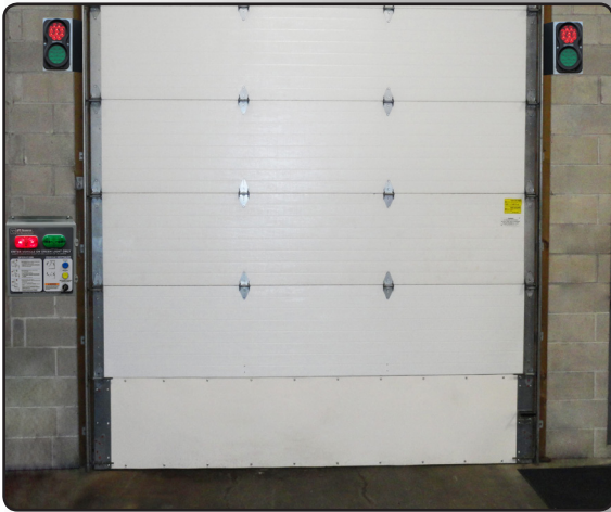
Aerial Safety Lights
