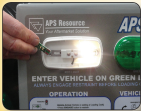
Inside LED Upgrade
