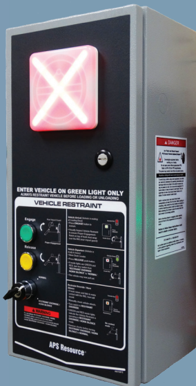
Figure 2: PLC-based control panel with red/green composite light
