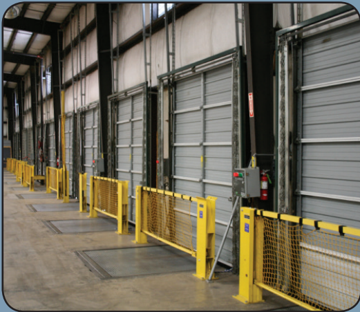
Figure 2: Multiple Dock Impact Barrier installations
