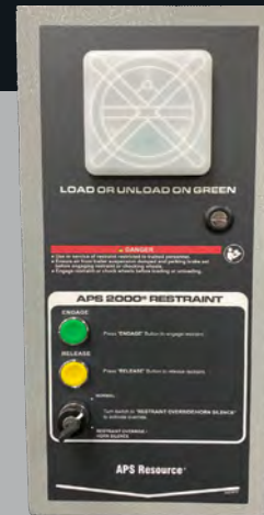
PLC-based control panel with red/green composite light
